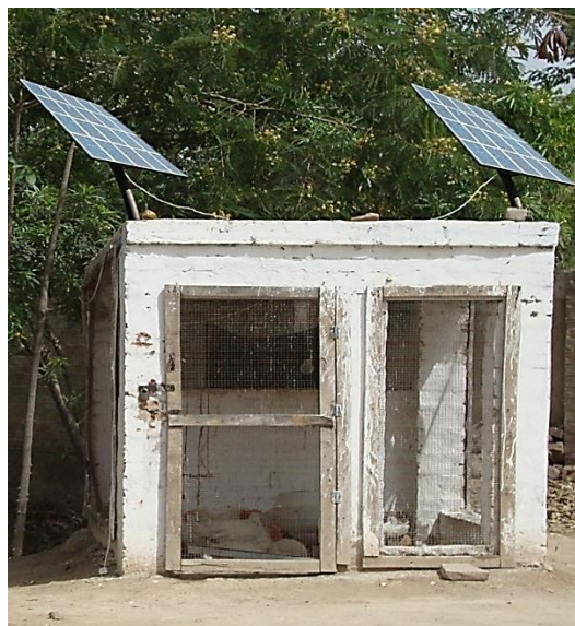
Figure 3: Solar electricity based poultry shed.
